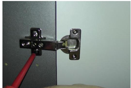
If, having loosened the backplate fixing screws, you find that the backplate refuses to move, you may need to give it little tap with a hammer. If it's a traditional style of plate, you should find there's plenty of adjustment in the backplate to allow it to move up and down. As with removing the doors, we suggest getting some help to support the weight of the door while you attach the hinges to the backplates.
