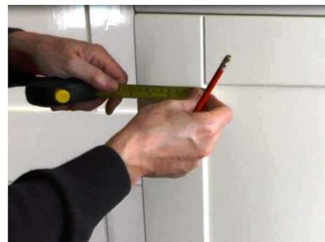
For example: if a door is 90mm, set up the drilling jig to allow you to drill a hole 55mm from the top of the door and half way in the centre of the door frame which is 45mm from the edge of the door.
